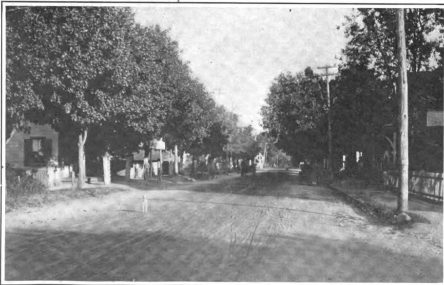
BEGINNING OF THE HICKSVILLE CONTROL—RAILROAD CROSSING IN THE BACKGROUND
